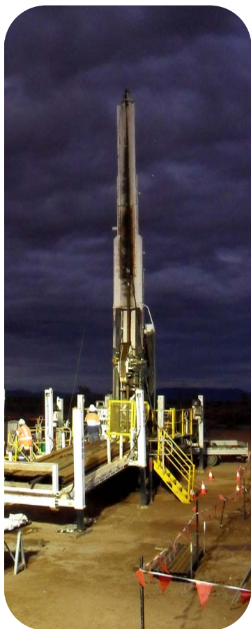
Boart Longyear drilling operations at Treebeard 1A, Parachilna Project.
