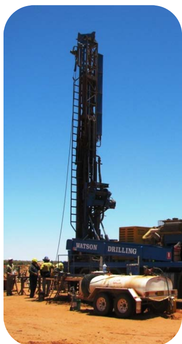
Watson Drilling diamond core drill rig during operations at Melkor 1
